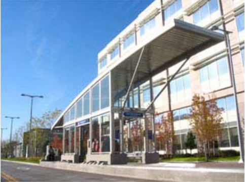
Cleveland Euclid Corridor Bus Rapid Transit Station
